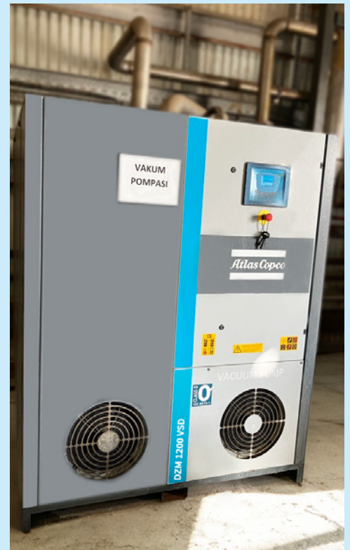
Noordzee facility with DZM 1200 VSD + pump
