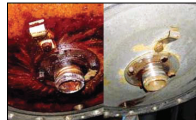
Vessel cover contaminated
