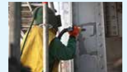
8.6 to 10 bar: Abrasive blasting
