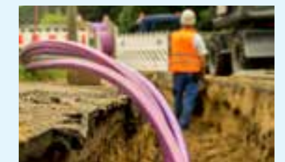
12 to 14 bar: Cable blowing and drilling
