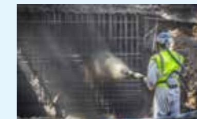
7 to 12 bar: Shotcrete applications
